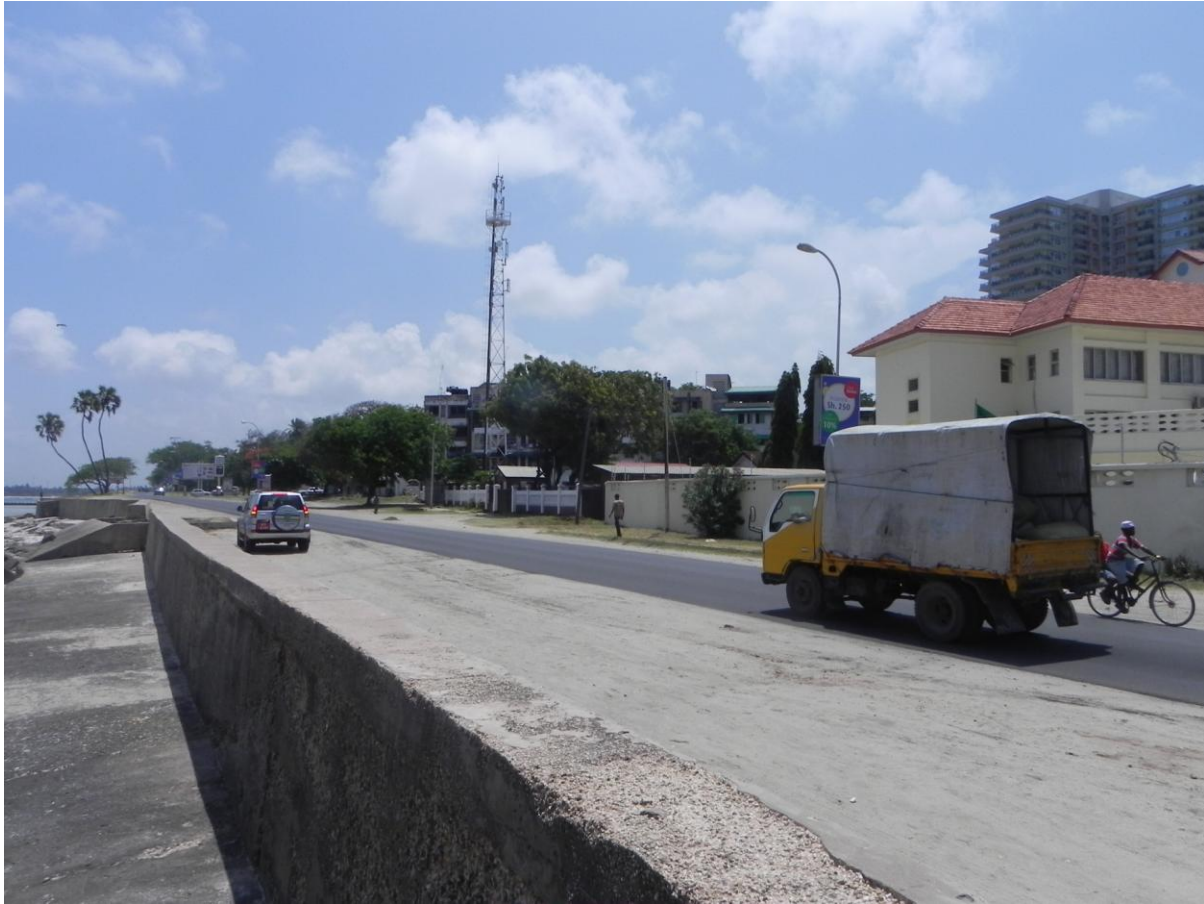
Figure 6: Relation of the current sea wall to Ocean road and other infrastructure Proposed rehabilitation of Dar es Salaam seawall at Ocean Road.
