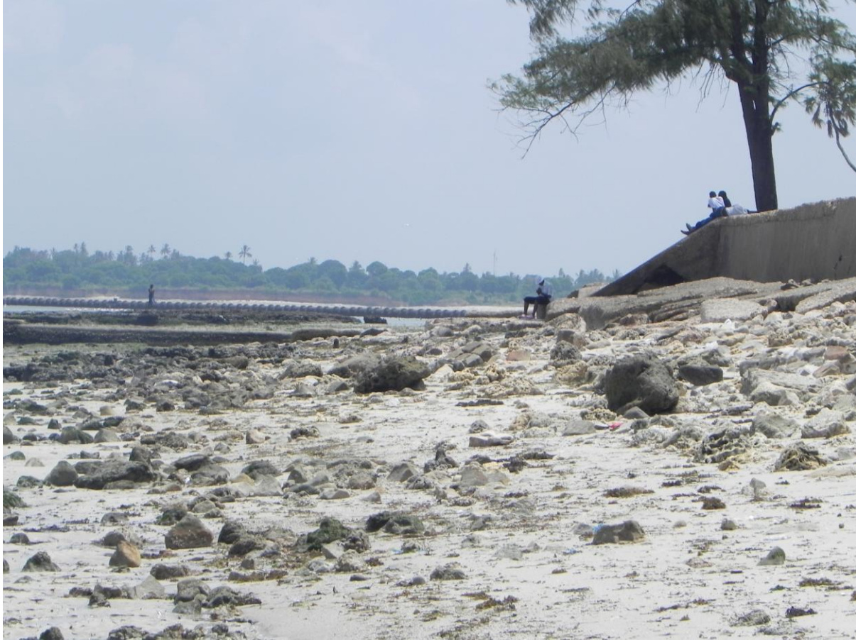
Figure 5: Evidence of water movement towards the wall
